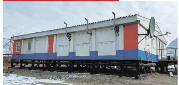
SAHPS Oymyakon. Power center
